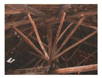
Figure 7: Elements of the roof timber structure over the apse of the Cathedral of Vercelli
