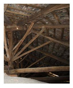
Figure 7: Elements of the roof timber structure over the apse of the Cathedral of Vercelli
