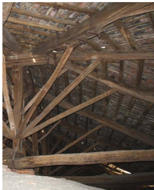
Figure 10 – Elements of the roof timber structure over the apse of the Cathedral of Vercelli Overall state of conservation
