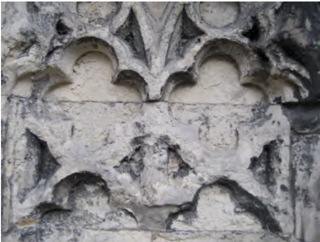
Figure 2: Detail of the surface blistering on the East wall.
