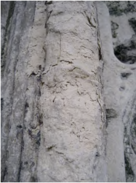
Figure 4: Macro photograph of flaking column on West wall.
