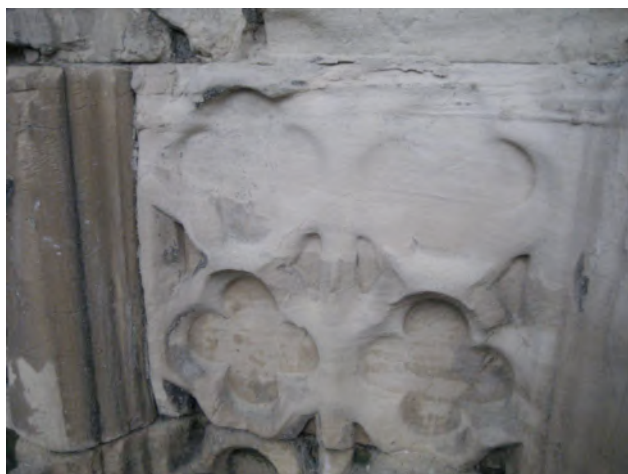
Figure 3: Detail of soft erosion on the North wall.
