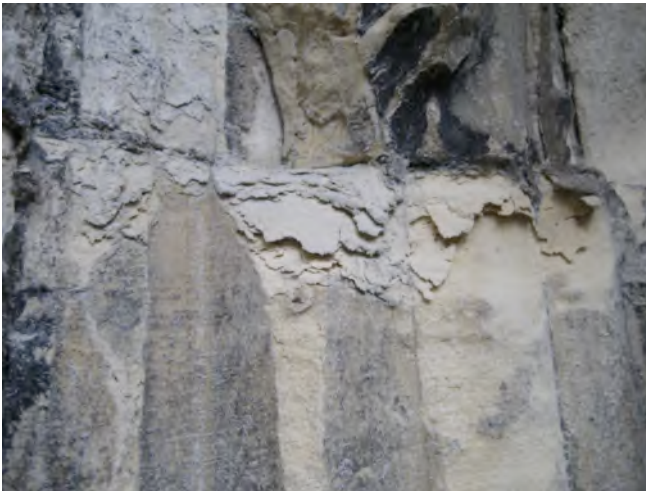
Figure 1: Detail of the flaking stone on the Northwest wall.
